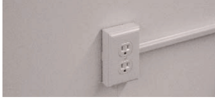
SURFACE WIRING CAN ALSO BE RUN HORIZONTAL IF THERE IS NO ELECTRICAL OUTLET IN THE JOIST/TRUSS CAVITY ASLL WILL BE INSTALLED IN.
