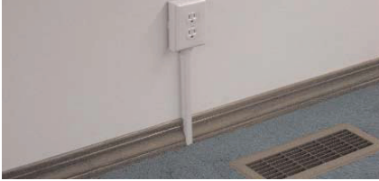
FINAL SURFACE WIRING INSTALLATION WITH ASLL.
