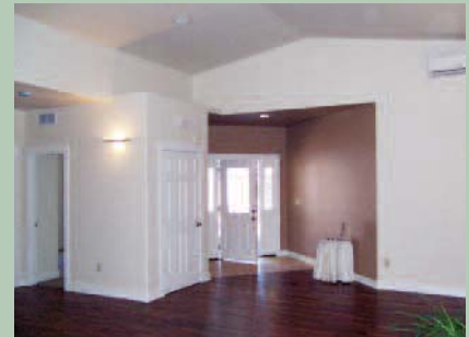
Photo shows AireShare™ blower grille above door on left and air handler for ductless split system at upper right corner.
